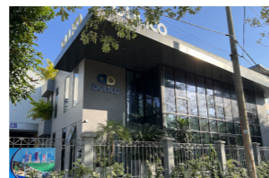
Headquarter & Factory 1: Lot A2, CN 7, Tu Liem Industrial Cluster, Nam Tu Liem, Hanoi, Vietnam
